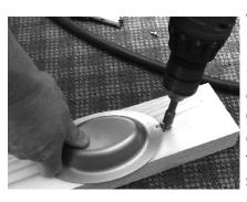
A 3/4" hole must be drilled into the handhole cover, near the center of the cover. Extreme caution must be used for safety reasons and to maintain the integrity of the cover during the drilling process. One example of the how to complete the drilling process successfully is to connect the cover to a scrap block of wood as shown. If the scrap wood method is not used, then the cover could spin and the sharp edges of the cover can cause bodily injury.
