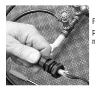
Find the electrical cord unit that is pre-assembled with the strain-relief mechanism on the exposed end.
