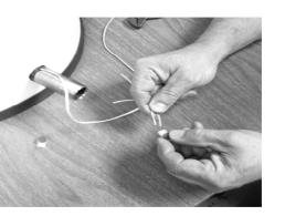
the red "UR" connectors found in the installation kit. The ends should already have been split apart approximately 1" (2.5cm). *The wire insulation does not need to be stripped, the "UR" connector will connect through the insulation.*
