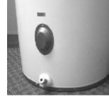
Locate drain valve at bottom of tank.
