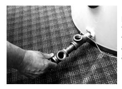
Now, insert the second brass "T" fitting, (item 103), onto the exposed end of the pipe, again leaving the "T" in the approximate vertical position.
