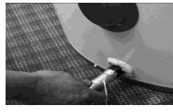
Once the drain valve is removed, apply thread seal tape to both ends of the 2" brass nipple, (item 102 (the one without the plastic tube), and install one end into the water tank where the drain valve was. This nipple has a temperature sensor attached to it. The nipple should be inserted
