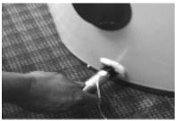
in the tank. On some electric tanks (such as Marathon) there will be obstructions within the tank due to the configuration of the piping within the tank. If the plastic in-feed tube does not enter the tank freely, please stop, and consult with a professional installer.
